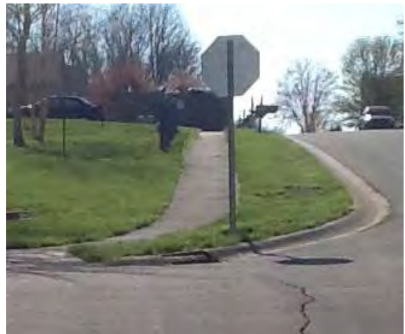
Example of +5% running slope following roadway grade
