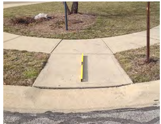
Example of good landing and turning space around street corner
